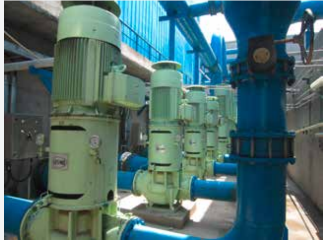
DESMI centrifugal pumps installed at Novozymes Tianjin plant.
